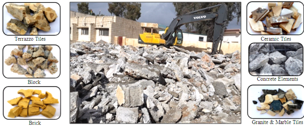
Figure (1) Demolished building of Al Rafidain bank in Koya city
